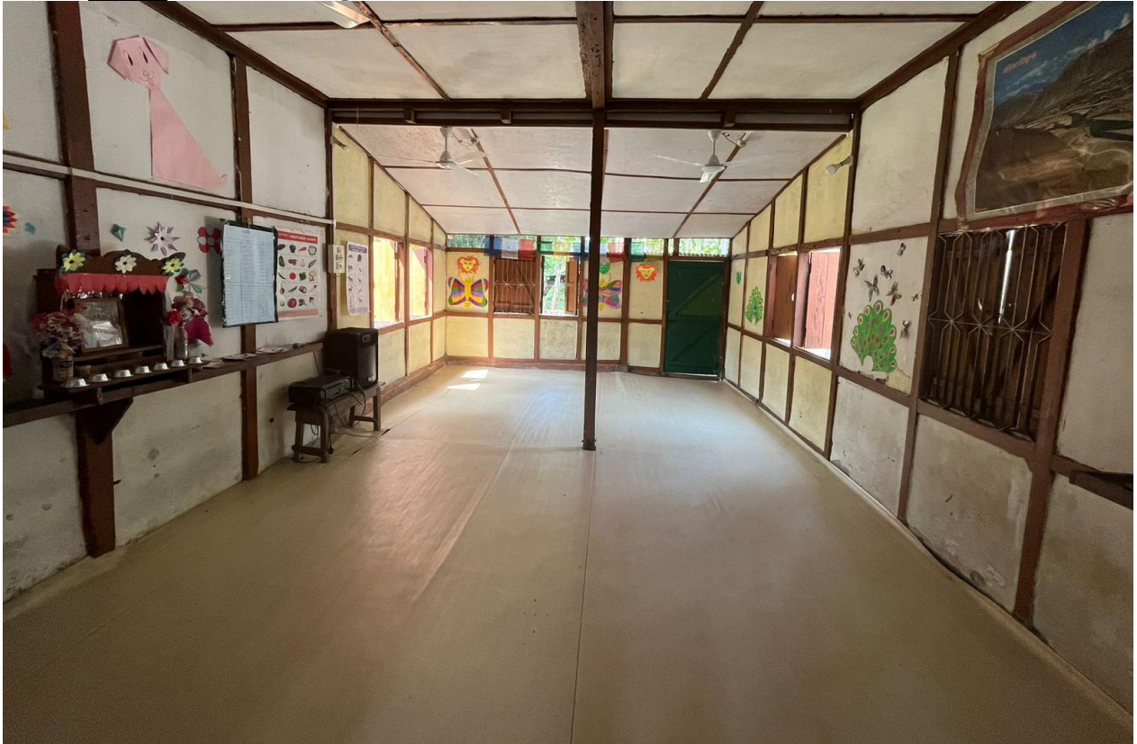
Photos before Hall window grill:
